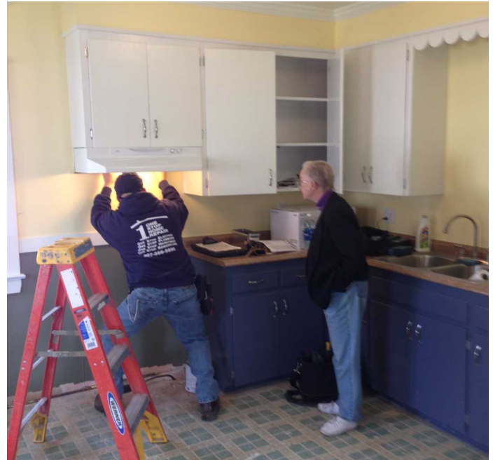
Our electrician installing a new light.
