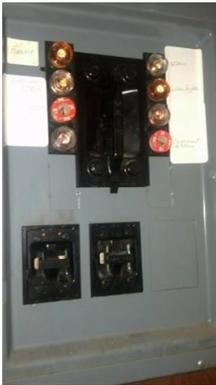
*A fuse box is not up to code. If your electric box looks like this, you should consider replacing it with breakers.*
